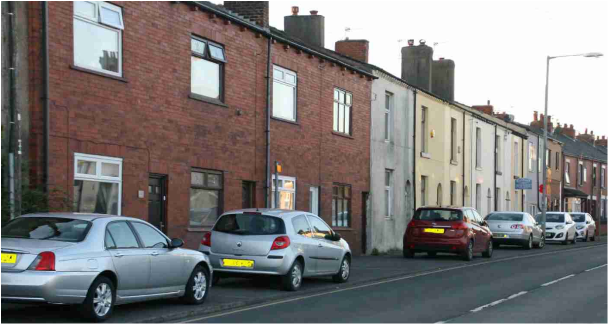
Pavement parking along New Street (current situation)
